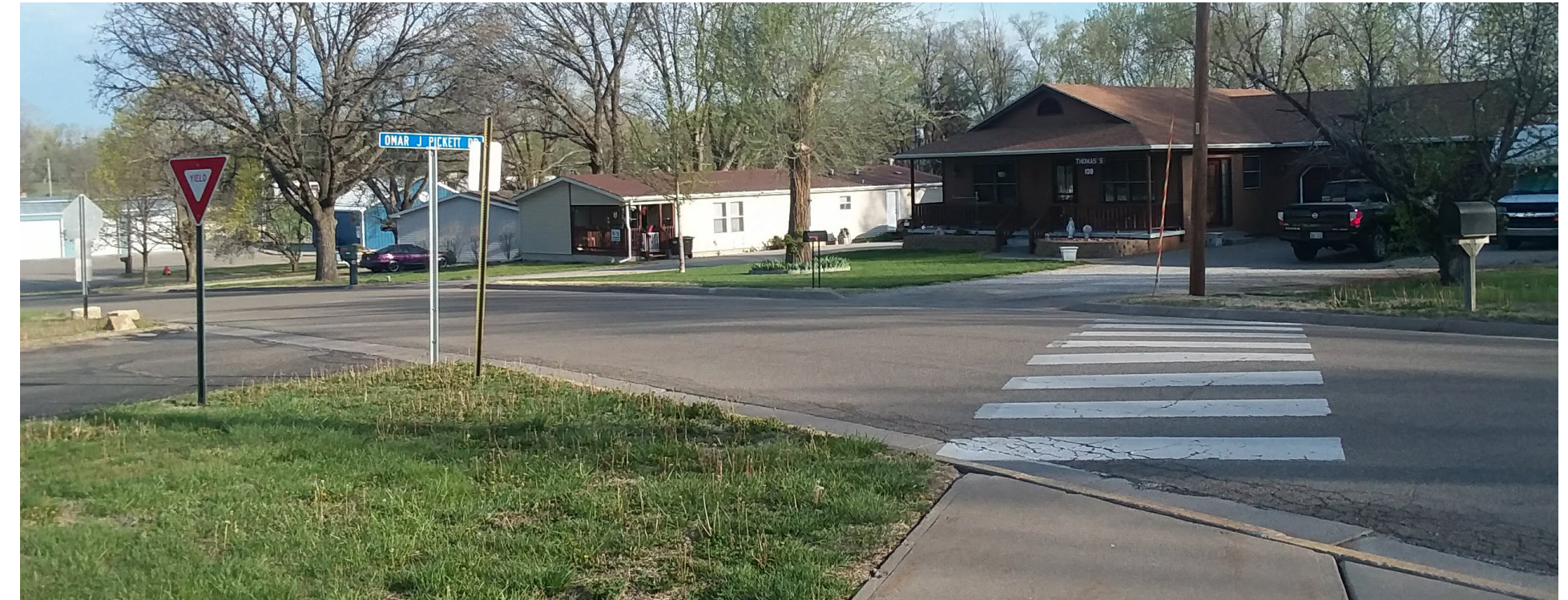
Figure 16: Grandview Elementary crosswalk
