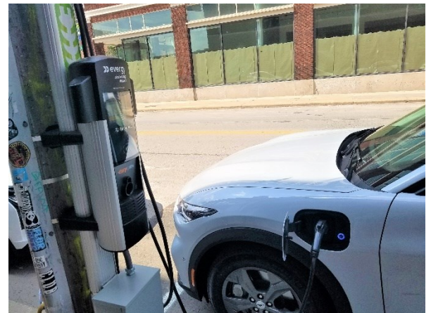
Figure 18. EV charger installation at 303 E. 18th St, Kansas City, MO 64108
