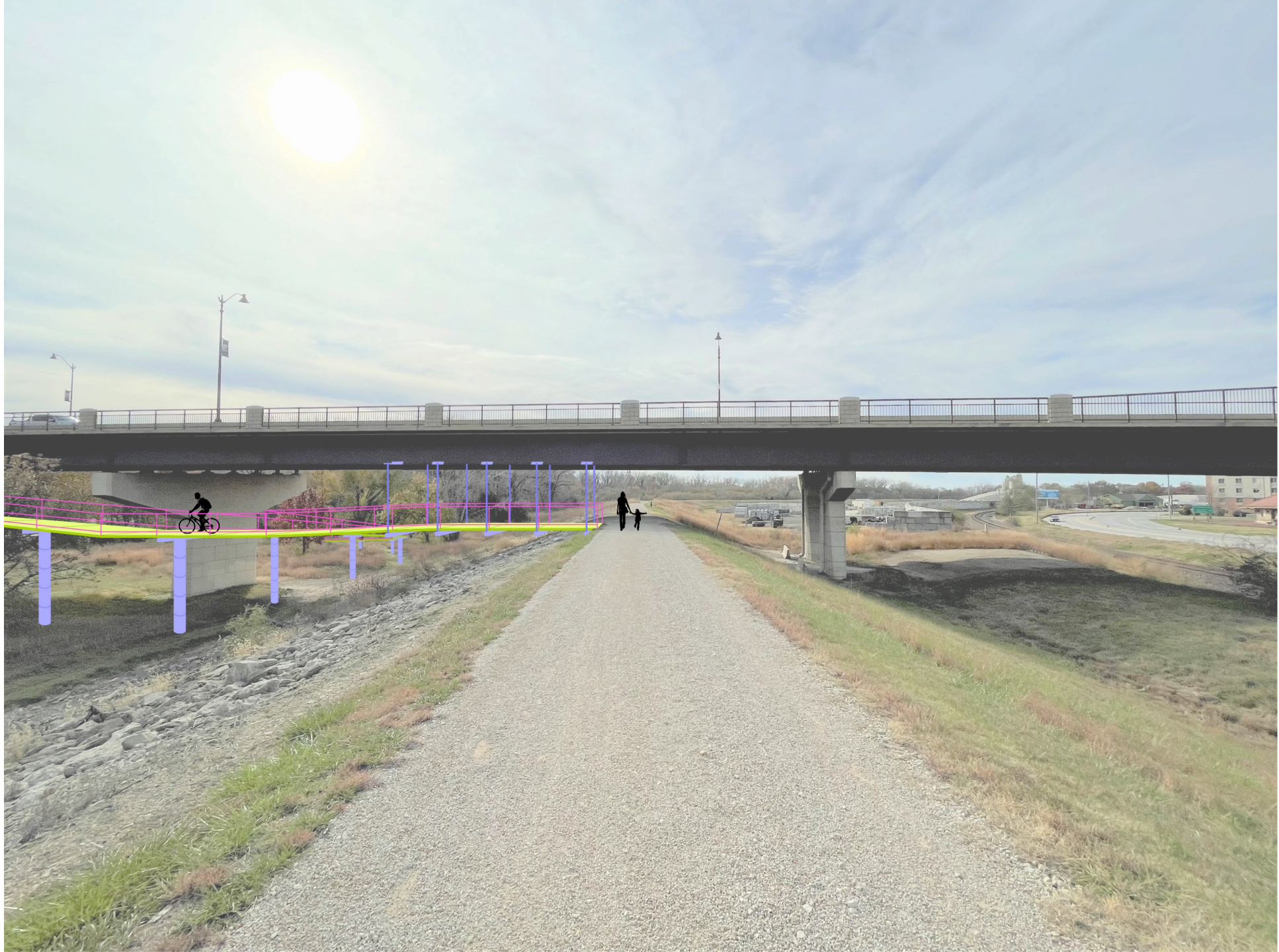
View of the Linear Trail and the junction with the K-177 bridge connector. Note, the suspended portion over the levee to remove impact the levee.
