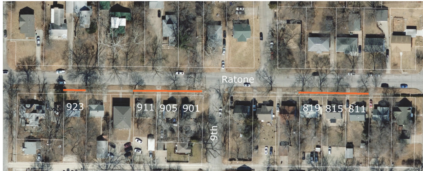
Figure B22. Poor-quality sidewalks along Ratone Street.
